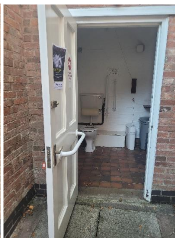
Entrance to Accessible toilet
